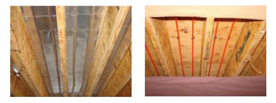
Paper backing, with and without out an aluminum foil reflective barrier was installed in portions of the project in order to assess the value of this method in reducing back losses.
