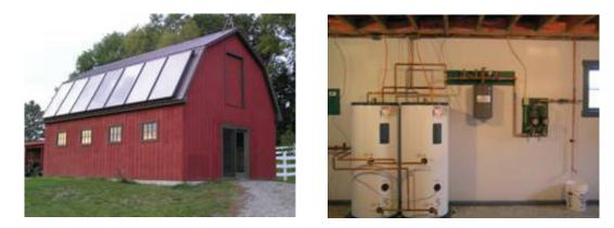
The testing facility was constructed of typical frame construction and was divided roughly in half in order to observe different tubing strategies under equal and identical conditions and make meaningful comparisons between the two without the issues of confounding variables. Heating performance is determined by very careful measurements of water flow and temperature measurements of the water going into and out of the systems.
